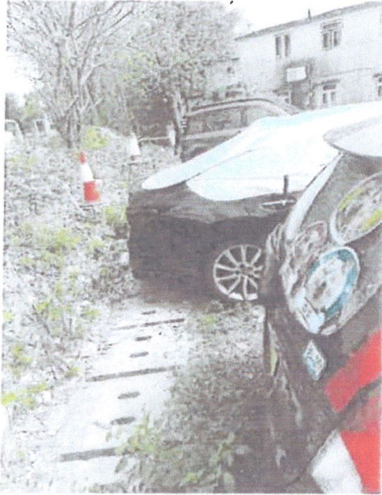
PHOTO NO. 3 Existing 700mm Covered Surface Channel Along Western Boundary of the Application Site
