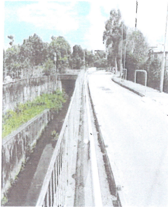
PHOTO NO. 1 Existing Open Rectangular Channel West of the Application Site
