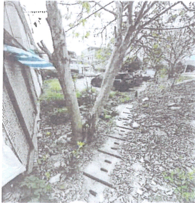
PHOTO NO. 2 Existing 700mm Covered Surface Channel Along Western Boundary of the Application Site
