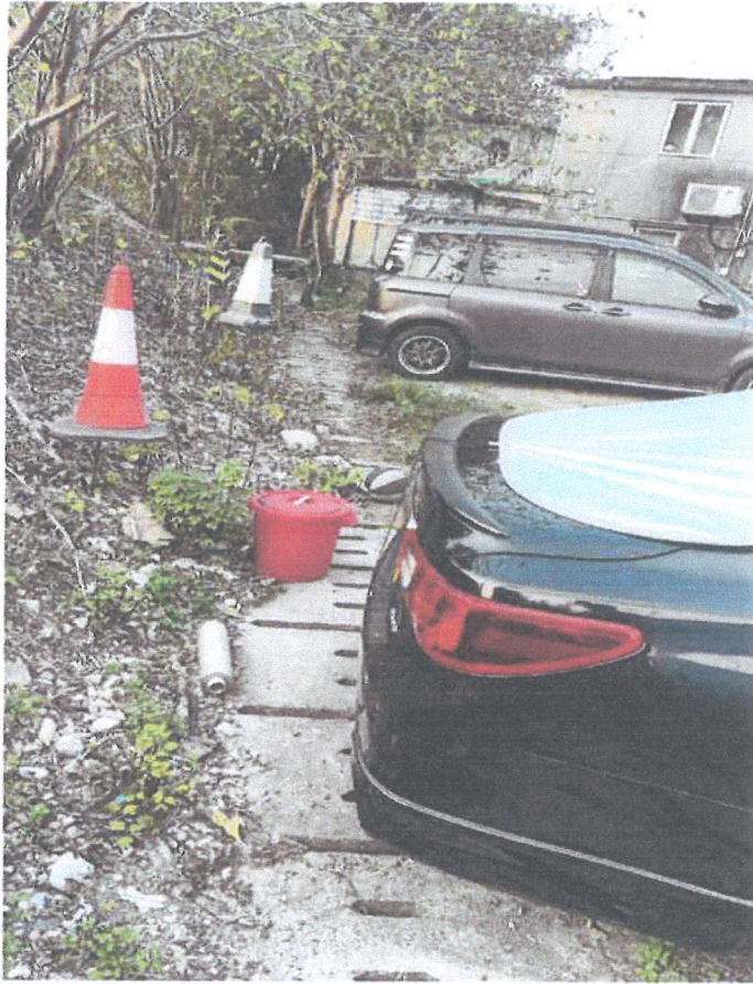
PHOTO NO. 6 (EXISTING 700MM U-CHANNEL)
